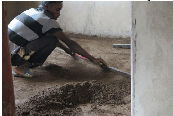
Preparing the floor in the new house for tiling
