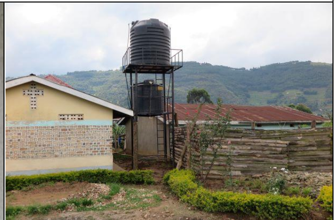
The elevated water tanks
