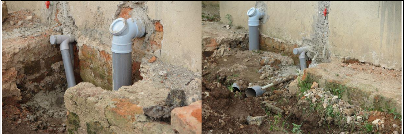
Plumbing work at the new house
