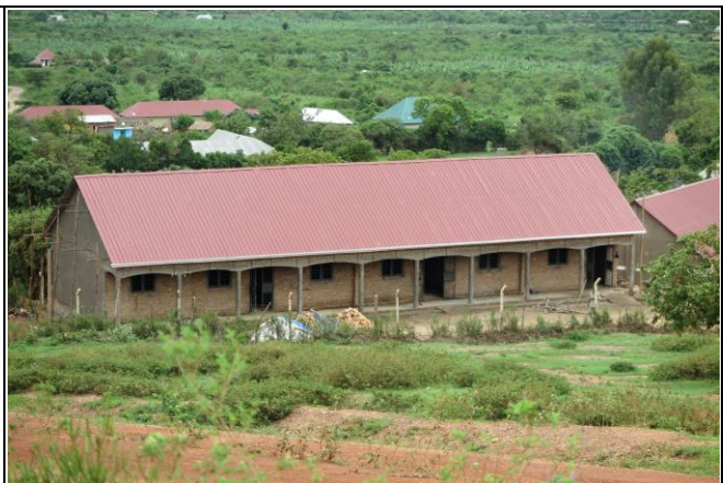
The construction of the new 3-classroom block is progressing
